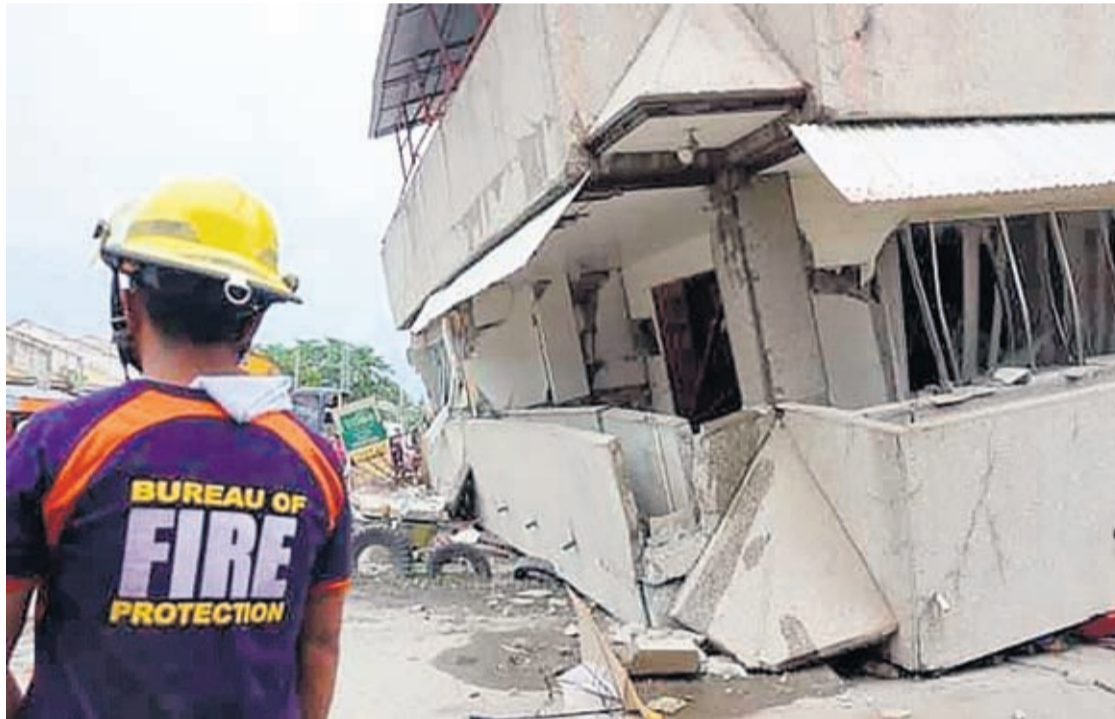
Rescuers check a collapsed building following an earthquake that struck Padada, Davao del Sur province, southern Philippines on Sunday Dec. 15, 2019.
